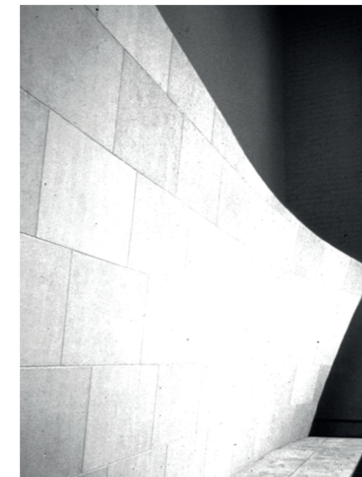
[Fig.1] Frank Gehry - Disney Concert Hall in Los Angeles[1] Pieces of stone are fabricated via three-axis milling. Complex shapes are realised using two novel methodologies: 3D CAD and three-axis CNC.
